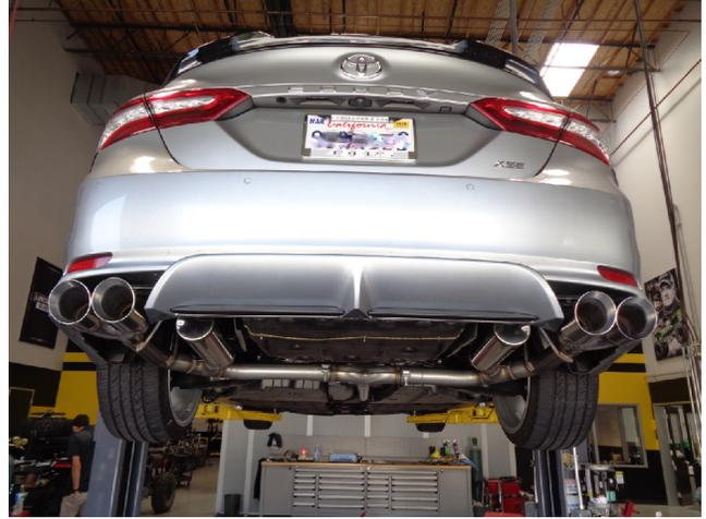
**Step 4.** Once a final position has been chosen for the new exhaust system, evenly tighten all clamps and fasteners, from front to rear, using the torque specifications on page one of the instructions. Inspect all fasteners after 25-50 miles of operation and re-tighten if necessary.
