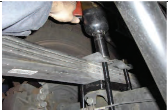
Raise axle, install new u-bolts and hardware, tighten.
