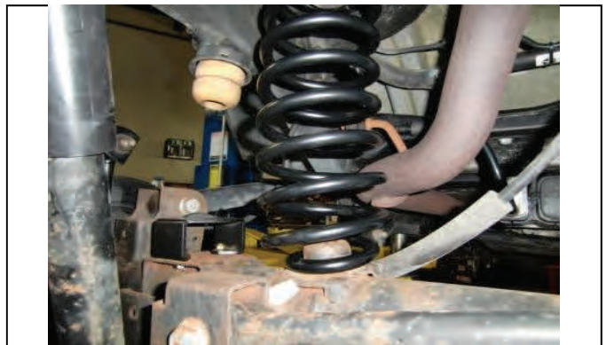
Install new coil springs and OE isolators and raise axle.
