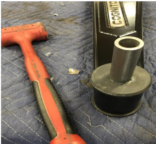
Figure 23: Install Crush Sleeve
