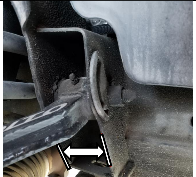
Figure 2: Factory Frame Service Perch Removal - After
