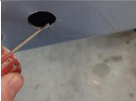
59. Use suitable rust preventative touch up paint to coat the exposed metal to prevent future rust.
